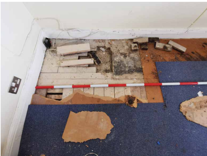
Plate 55: Residence 15; ground floor; Office room 3 - floor
