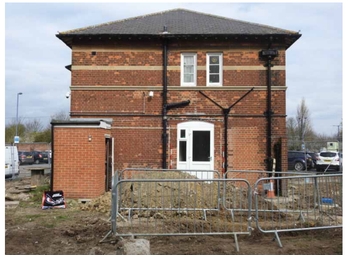
Plate 42: Residence 15; South-south-east elevation
