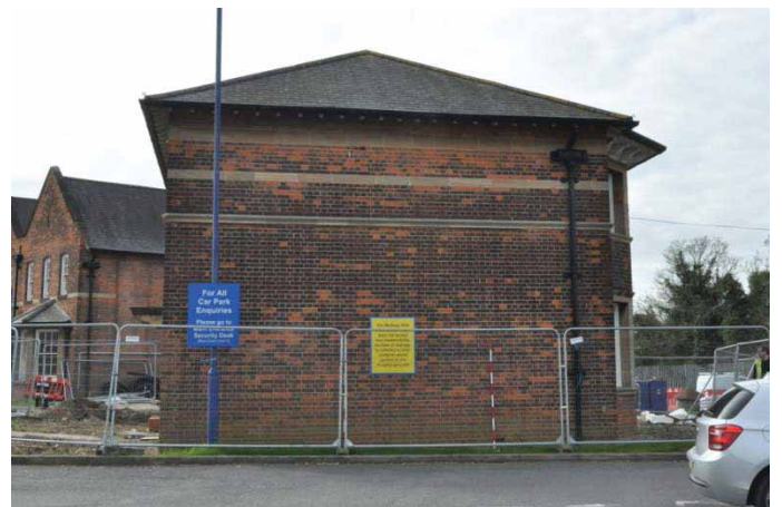
Plate 44: Residence 15; South-south-east elevation
