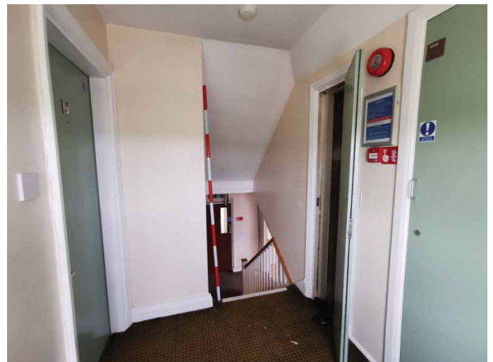
Plate 35: Residence 14; Second floor – Bedroom no. 12 on the left and tank room on the right
