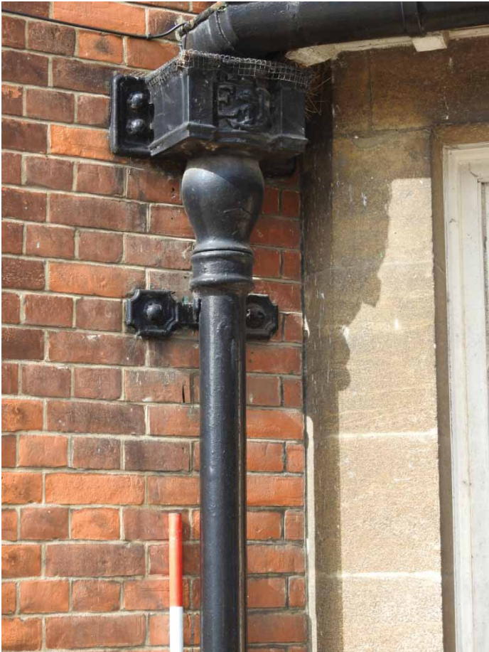
Plate 10: Residence 14; NE elevation; Looking west at bay window gutter box
