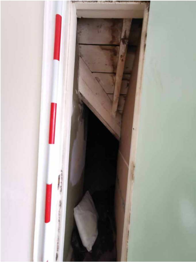
Plate 36: Residence 14; Second floor – compartment with exposed roof beams located behind tank room
