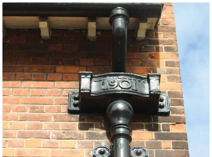
Plate 17: Residence 14; SE elevation; NE end - gutter box
