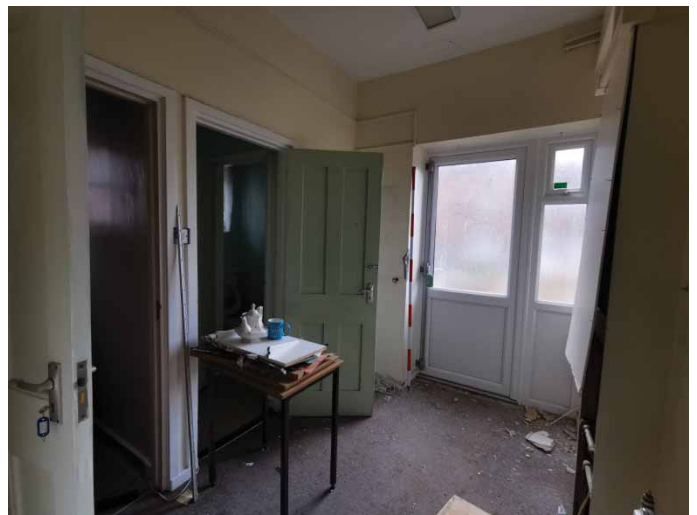
Plate 56: Residence 15; ground floor; Side entrance and WC and store on the left
