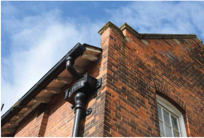
Plate 12: Residence 14; NE elevation; Looking west at roof eaves
