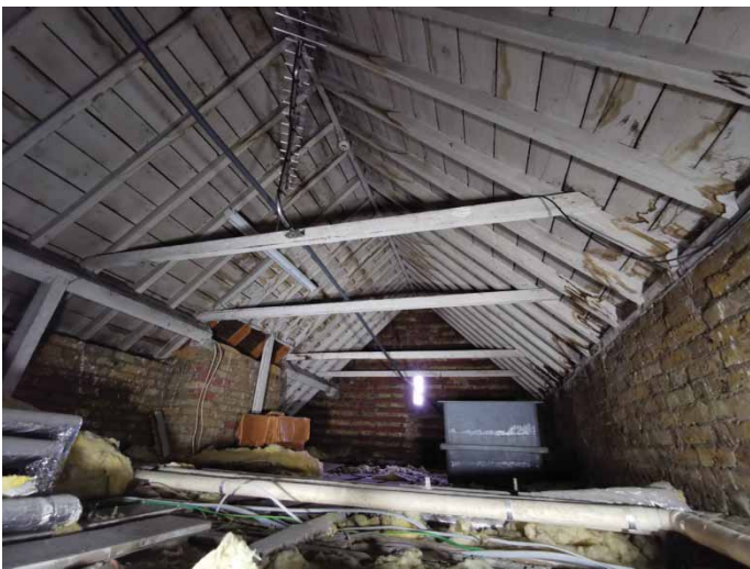
Plate 38: Residence 14; Looking SW at the roof beams
