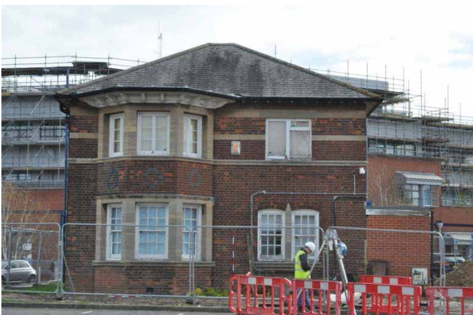
Plate 43: Residence 15; West-south-west elevation
