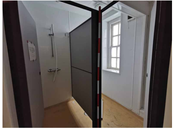
Plate 25: Ground floor; shower and toilet unit
