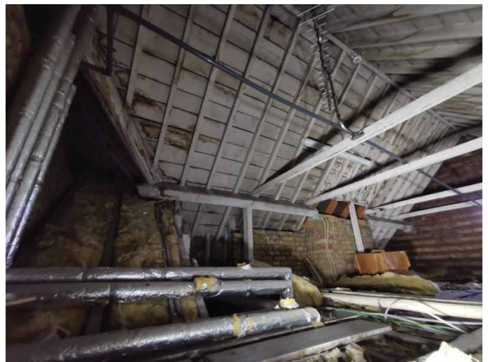
Plate 39: Residence 14; Looking SW at the roof beams
