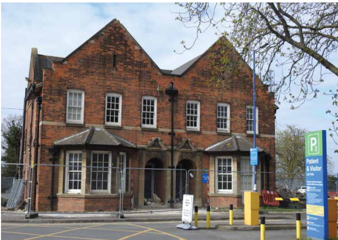
Plate 4: Residence 14; North-east elevation
