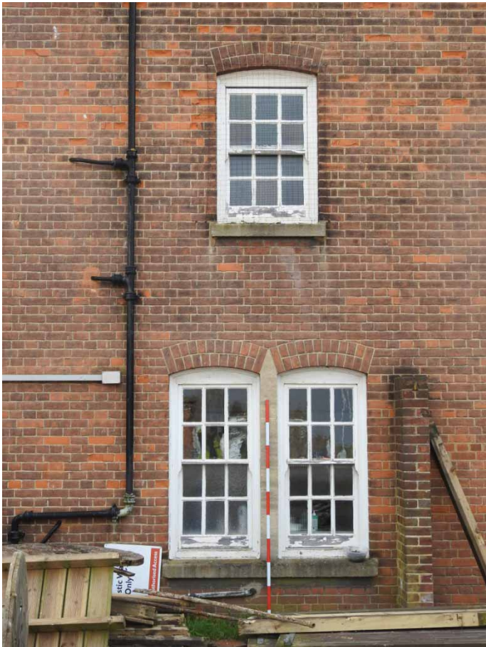
Plate 14: Residence 14; SE elevation; 1 st and ground floor windows
