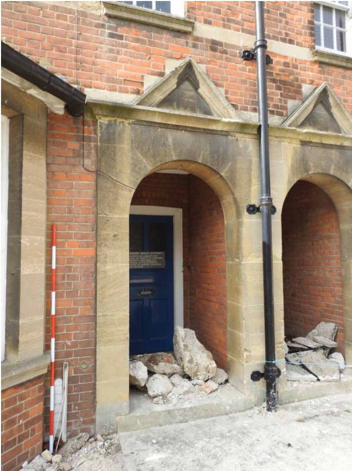
Plate 8: Residence 14; NE elevation; Portico entrance
