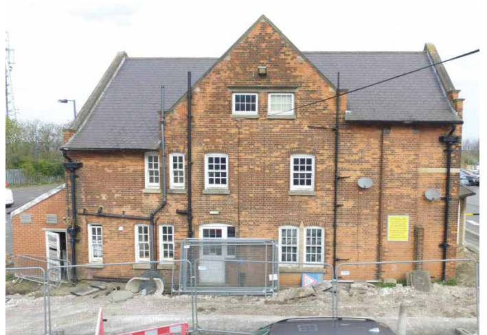
Plate 5: Residence 14; South-east elevation
