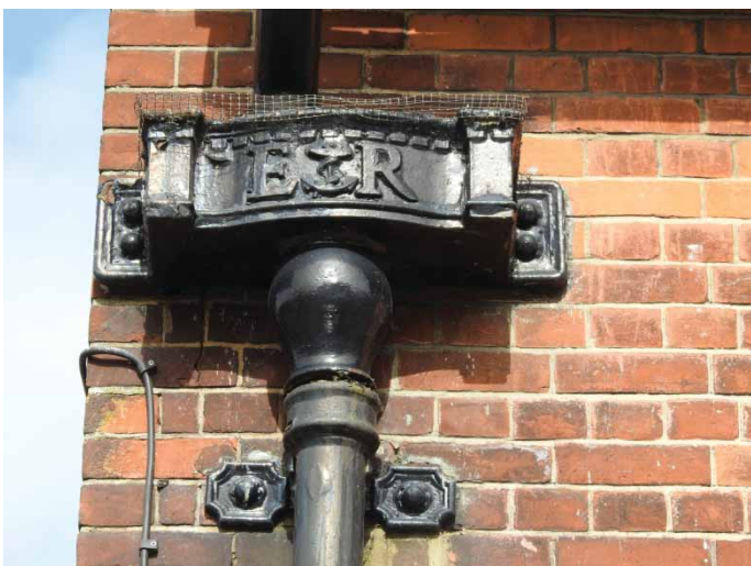
Plate 16: Residence 14; SE elevation; SW end - gutter box
