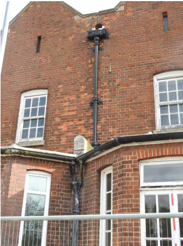
Plate 20: Residence 14; SW elevation; gutter
