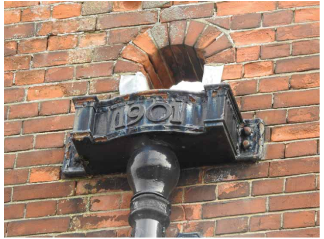
Plate 19: Residence 14; SW elevation; gutter box
