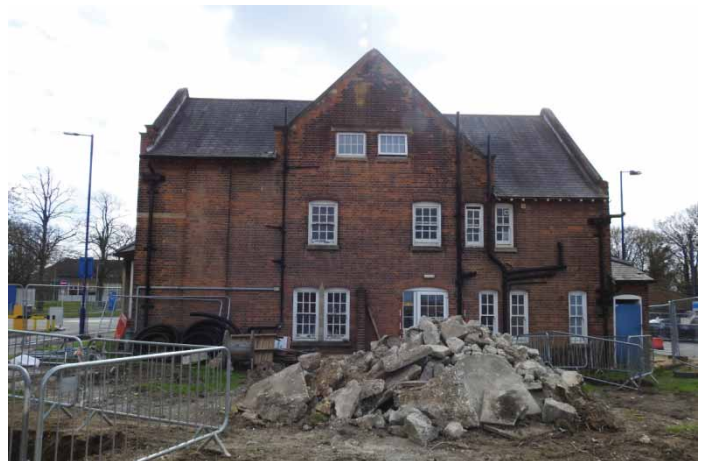
Plate 7: Residence 14; North-west elevation
