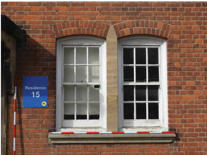
Plate 47: Residence 15; ENE elevation, windows
