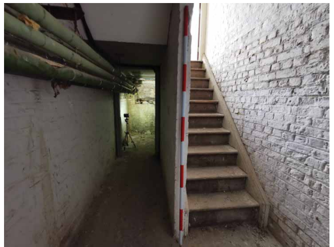
Plate 23: Residence 14; Basement and stairs to the ground floor
