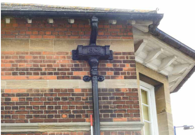
Plate 49: Residence 15; SSE elevation, Roof eaves and gutter box
