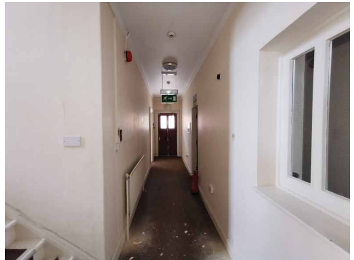
Plate 27: Residence 14; Upper ground floor – corridor and main entrance door
