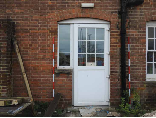
Plate 18: Residence 14; NW elevation; entrance doorway
