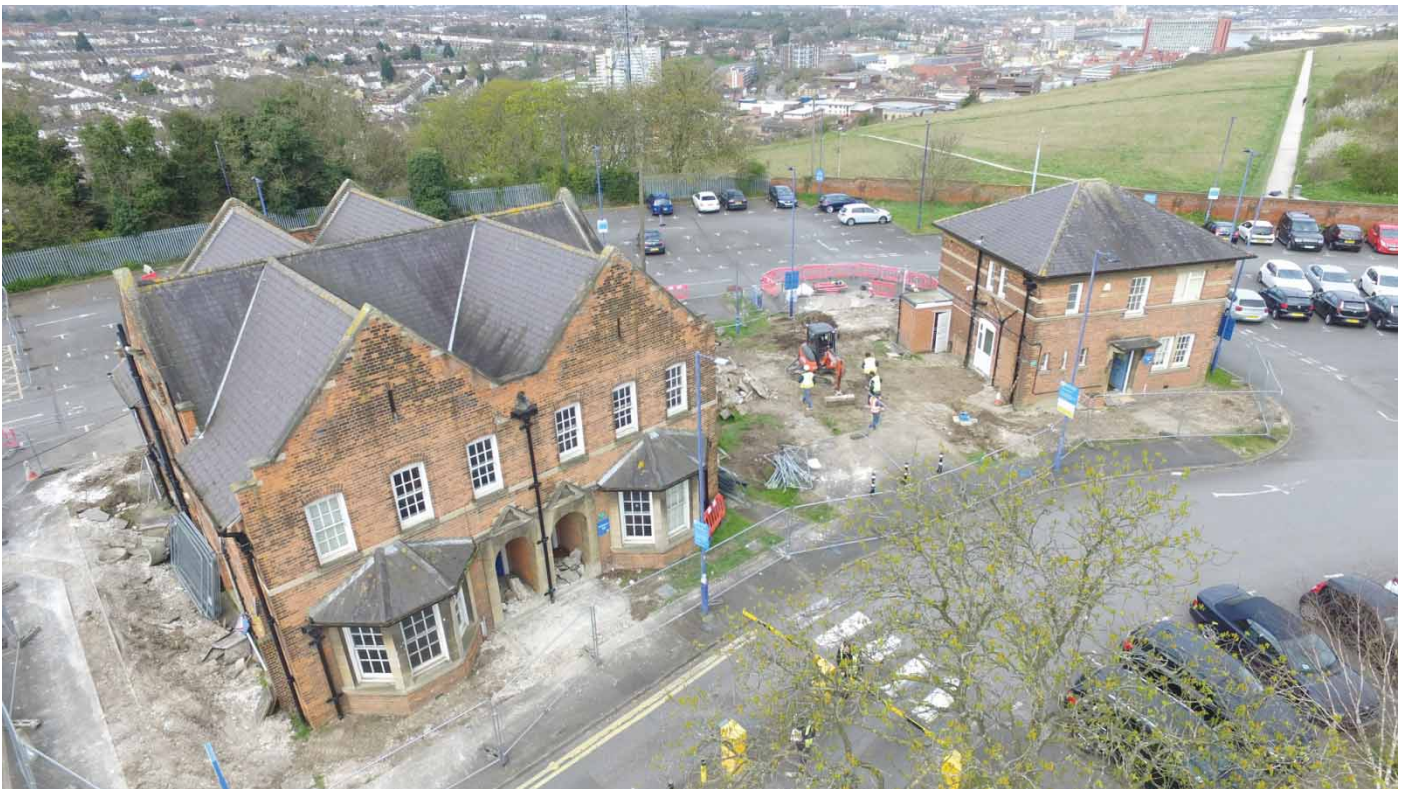
Plate 2: Looking west at the buildings; Residence 14 on the left and Residence 15 on the right.
