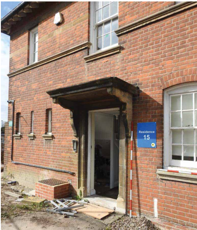
Plate 45: Residence 15; ENE elevation, Looking SSW at main entrance
