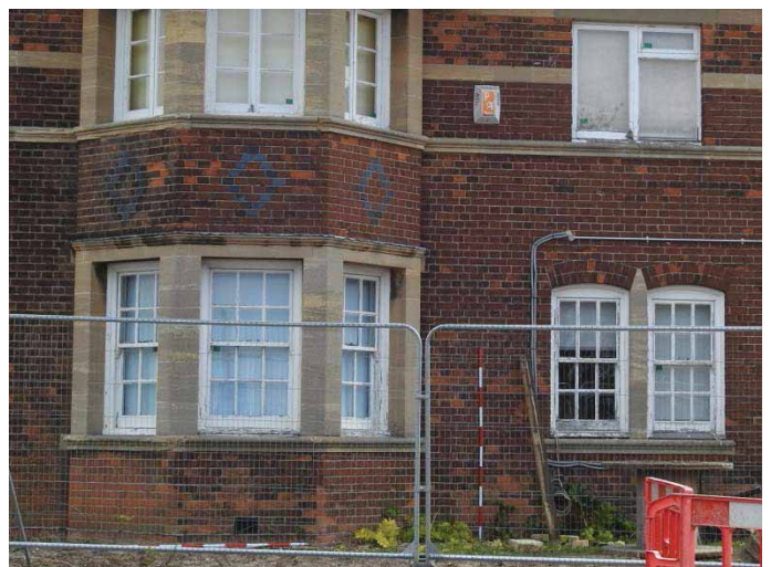
Plate 50: Residence 15; WSW elevation, windows
