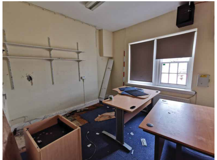
Plate 54: Residence 15; ground floor; Office room 3
